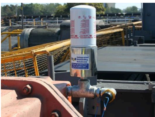
Figure 2 – Breather splash guard and assembly in use
